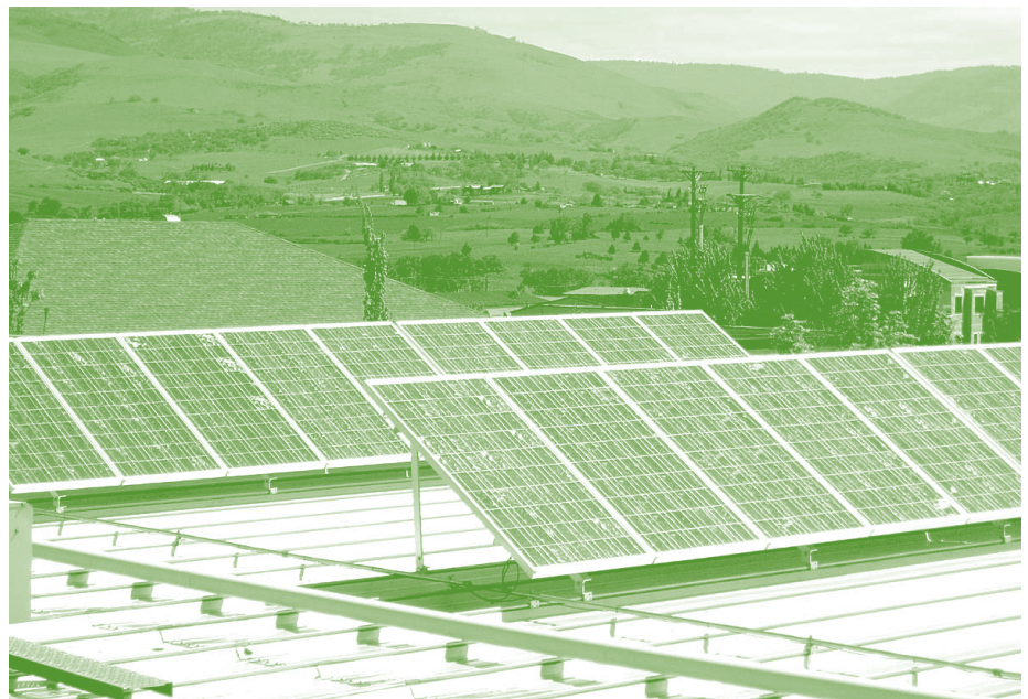
Solar panels basking in the sunshine.
